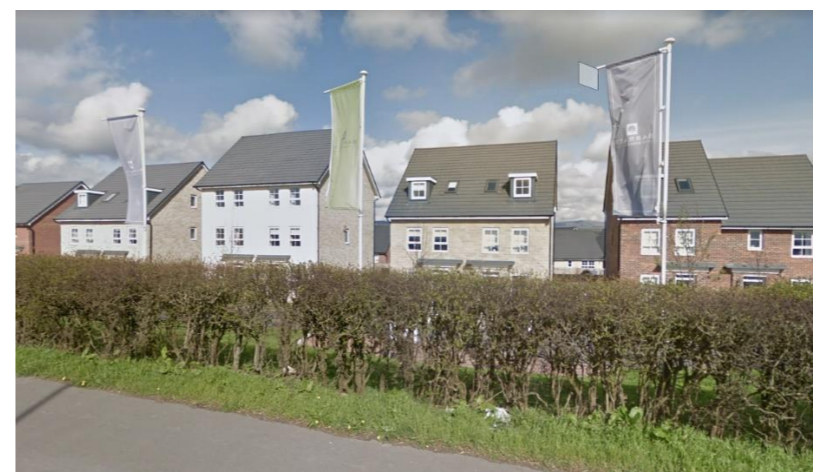
15. New 2.5 & 3 storey housing to the east of the site
