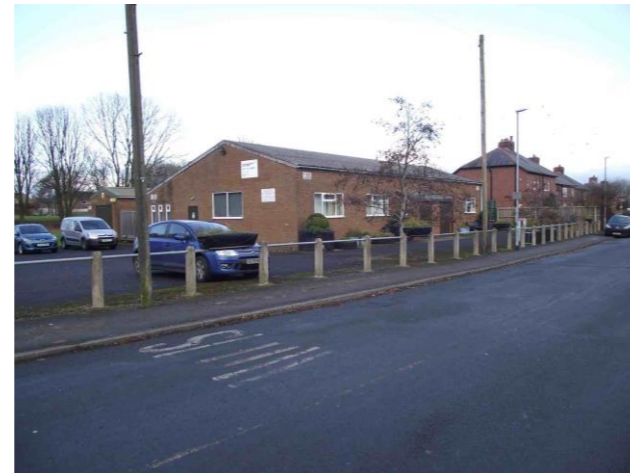
18. Scout Hut to Kepple Lane
