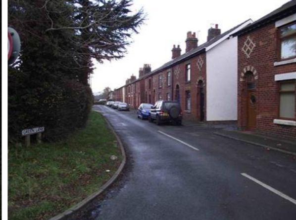
7. Terraced housing to Green Lane
